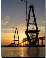
The bridge's 1,546-ft main span is supported by two 575-ft-high, diamond-shaped towers Source: constructoragc.construction.com
