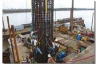
Insertion of rebar cage and O-cell assembly
