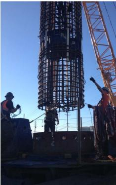
Reinforcement cage installation with O-cells
